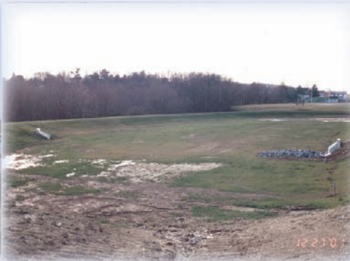
Stormwater detention basin
