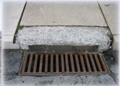
Storm drains are the common stormwater conveyance system in urban areas
