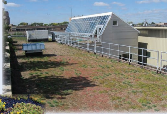
Above: Green roof installed on a flat roof
