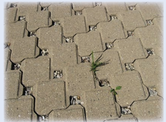
Pavement blocks allow precipitation to infiltrate into groundwater supplies rather than runoff
